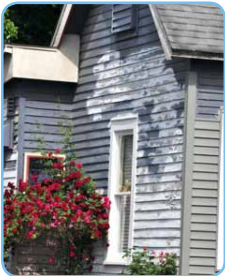
Many homes are in various stages of repair.
