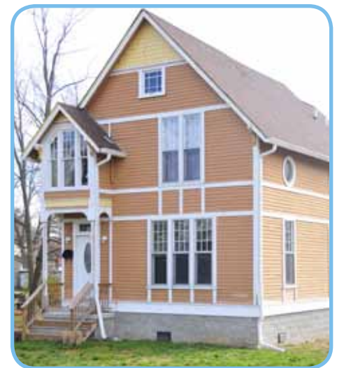
This restored home is in an area devastated by the 2008 flood. The raised foundation will help reduce the potential of damage in another flood event.
