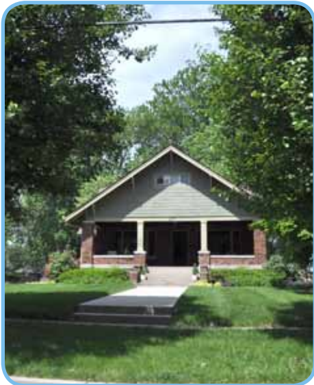
Traditional bungalows can be found throughout Franklin's core neighborhoods.
