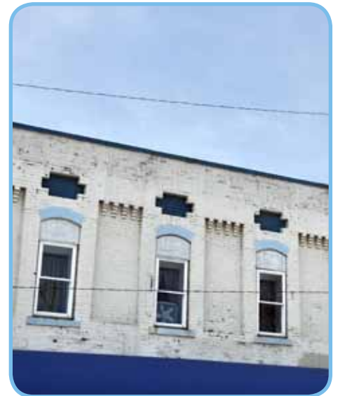
Second floor apartments over downtown businesses are an example of a mixed-use development.
