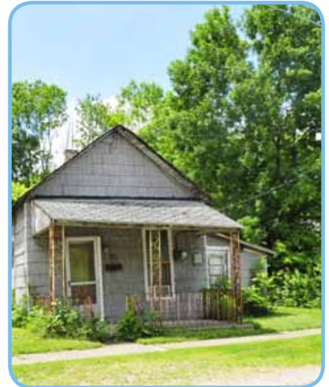
The homes on Johnson Avenue vary greatly in size and condition.
