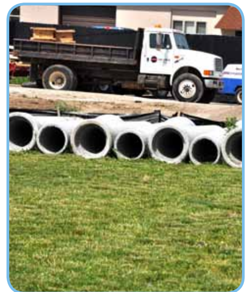
Recent improvements to downtown drainage systems.
