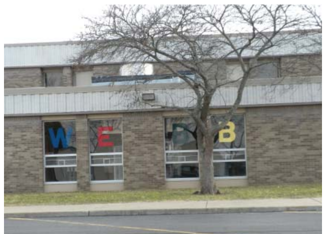
● WEBB ELEMENTARY SCHOOL - Source: HWC Engineering
