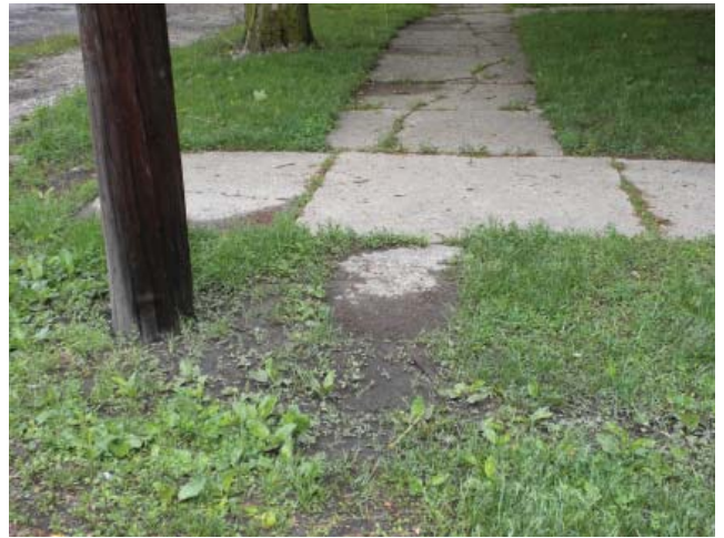
● Existing sidewalk repair issues - Source: HWC
