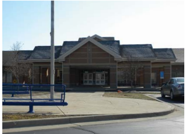
● CUSTER BAKER INTERMEDIATE SCHOOL - Main Entrance Source: HWC Engineering
