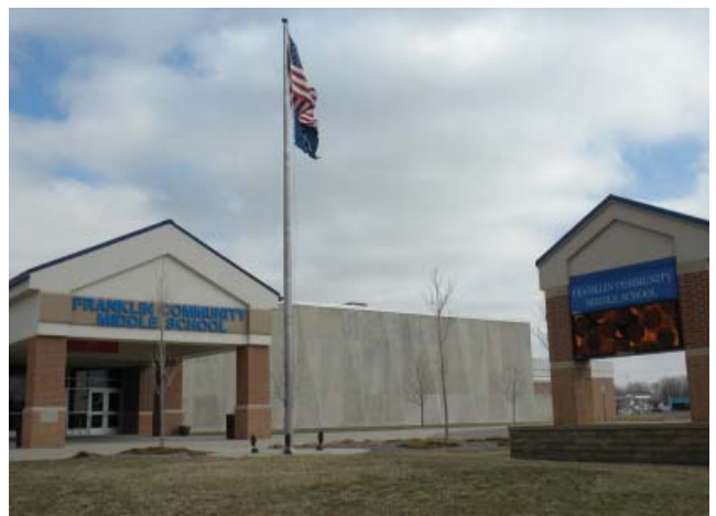
● FRANKLIN COMMUNITY MIDDLE SCHOOL - Main Entrance Source: HWC Engineering
