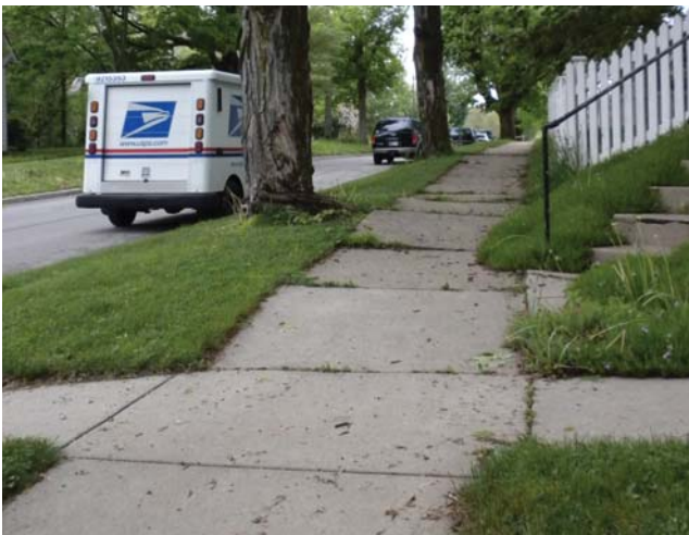
● Walnut Street - Sidewalks in need of repair/replacement. Source: HWC Engineering
