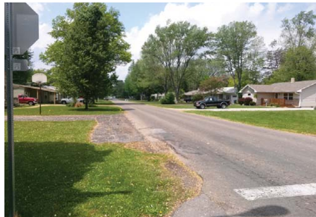
● Potter’s Green Neighborhood - Lack of Sidewalks Source: HWC Engineering
