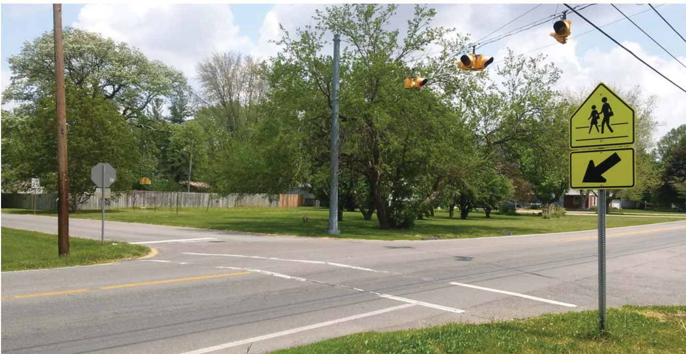
● Jefferson Street Intersection - Source: HWC
