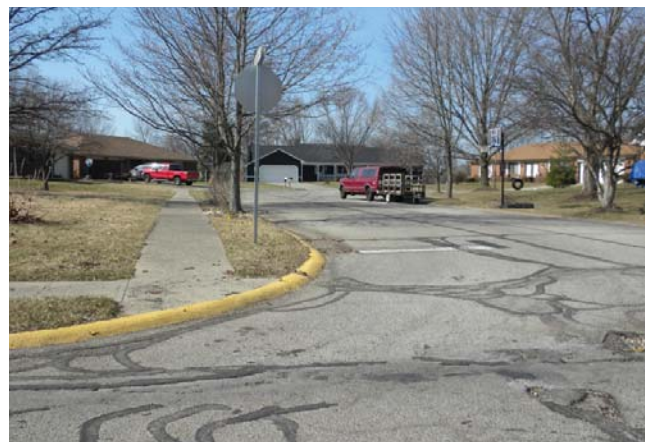
● Camelot Neighborhood - Non-compliant ADA Standards Source: HWC Engineering
