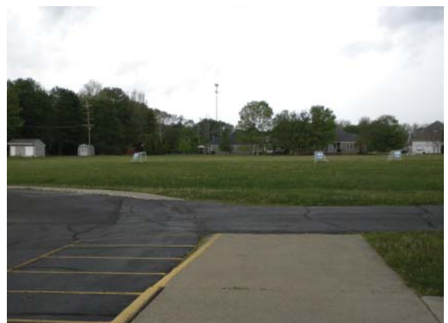
● WEBB ELEMENTARY SCHOOL - Existing sidewalks in need of repair on south side of school. Source: HWC Engineering
