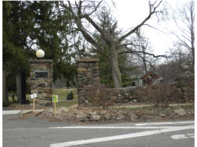
● Province Park Source: HWC Engineering
