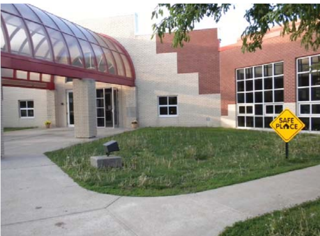
● NEEDHAM ELEMENTARY SCHOOL - Main Entrance Source: HWC Engineering
