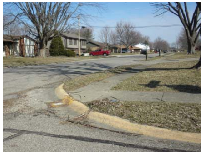
● Existing sidewalk curb transition issues - Source: HWC
