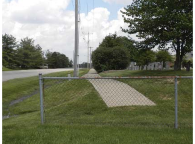
● Barrier for existing sidewalk - Source: HWC
