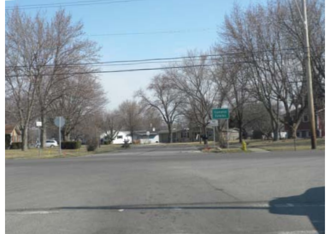
● CUSTER BAKER INTERMEDIATE SCHOOL - Existing intersection of Jefferson Street and Tracy Miles Blvd. Source: HWC Engineering
