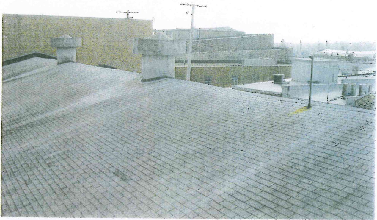
Photo 47 - The roof has an undulating appearance . . .
