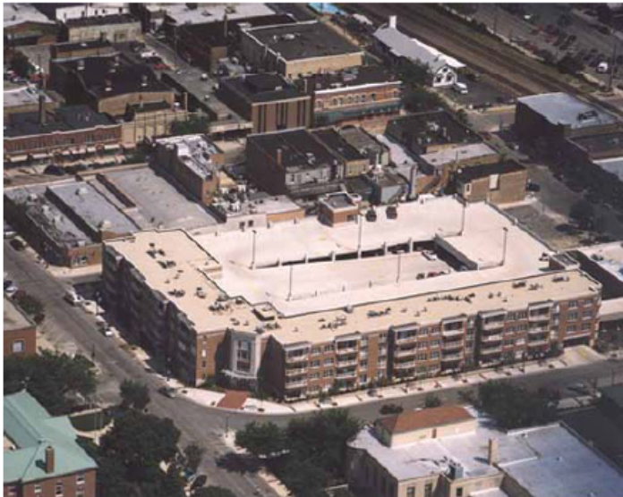
Wheaton Park Place Garage (Illinois)
