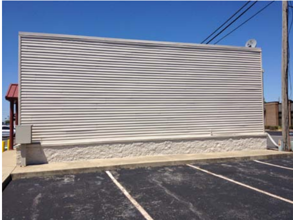
South Side Façade
