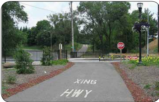
Greenway crossing at a highway. Source: nokenews.com.
