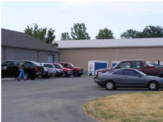
215 Industrial Drive – Front
