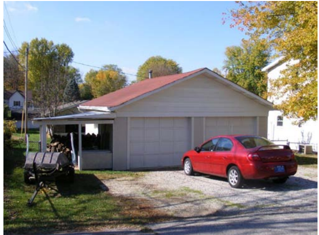
101 Pitt Street – Garage
