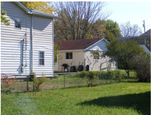
101 Pitt Street – Rear Yard/West Side
