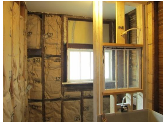
Insulation being added to the restroom.
