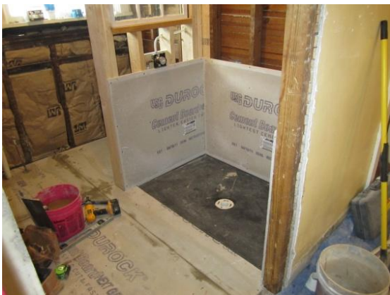
The beginning stages of installation of a handicap Accessible shower.
