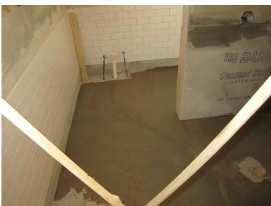
The beginning stages of installation of a handicap Accessible shower.
