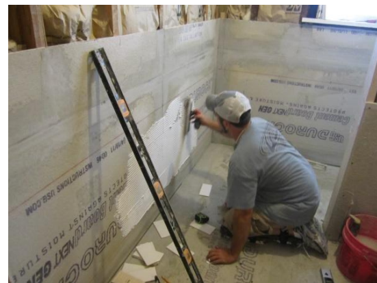
Sheet rock being prepped for subway tile.
