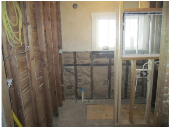
Restroom under renovation at 49 E. Madison Street.
