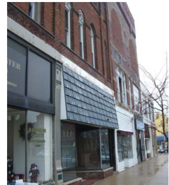
Inappropriate materials and use of Mansard roofing
