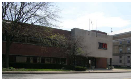
Not Recommended: horizontal window alignment with no windows in entrance
