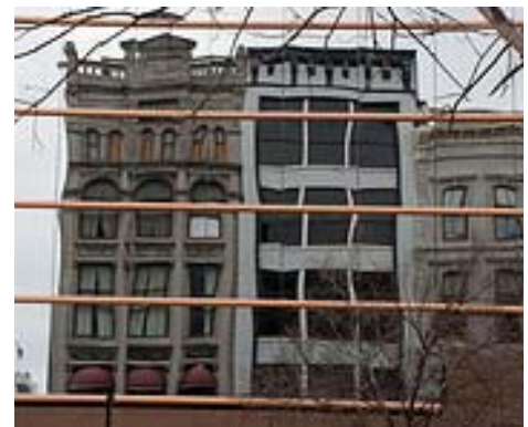
Not recommended: Inappropriate grillwork (above) and mirror glass front below
