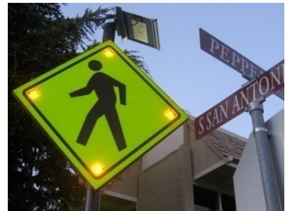
Pedestrian crossing signal with solar-powered lighting
