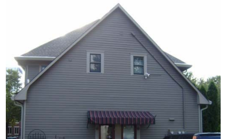
Above, roof line trim board inappropriately boxed in at bottom, Below, done appropriately
