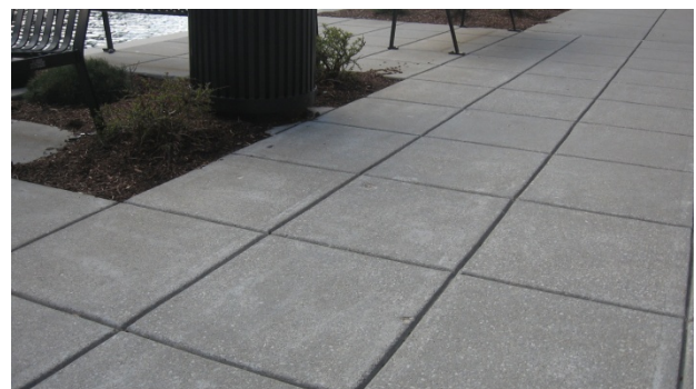
Urban trail example: cast-in-place concrete path with decorative score pattern
