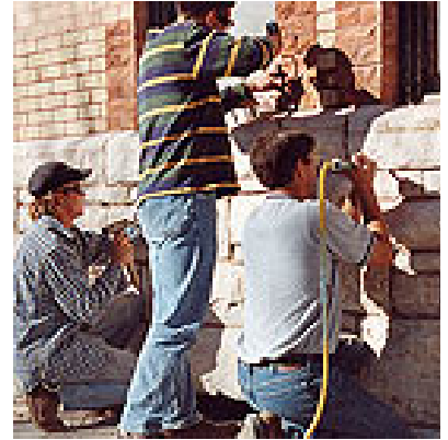
Careful & appropriate preparation of mortar joint – courtesy of Abstract Masonry Restoration
