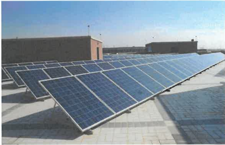
Figure 21. Rooftop mounted photovoltaic array
