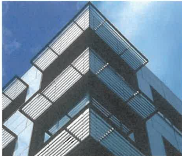
Figure 20. Integrated sunshading devices
