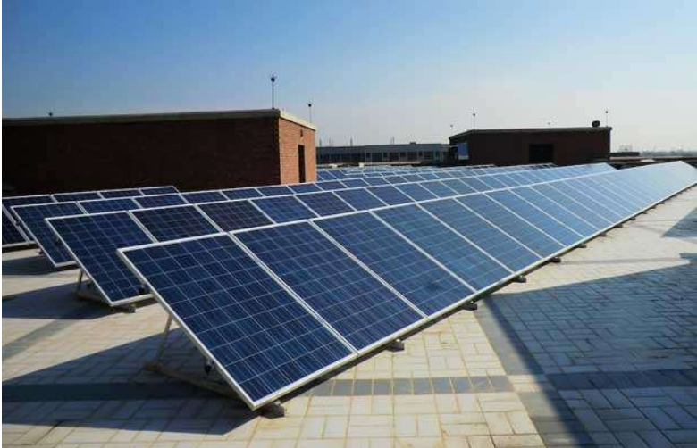
Figure 21. Rooftop mounted photovoltaic array
