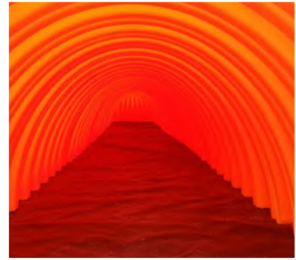
Looking down the Isolator Row from the manhole opening, woven geotextile fabric is shown between the chamber and stone base.
