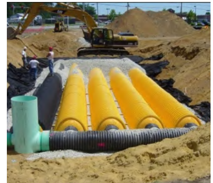
Looking down the Isolator Row from the manhole opening, woven geotextile fabric is shown between the chamber and stone base.
