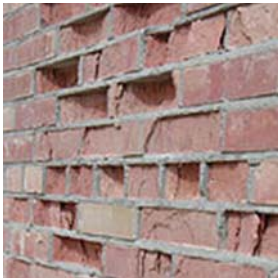
Excessively deteriorated brick
