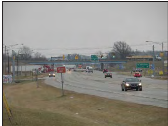
View looking east towards the interchange along King Street.
