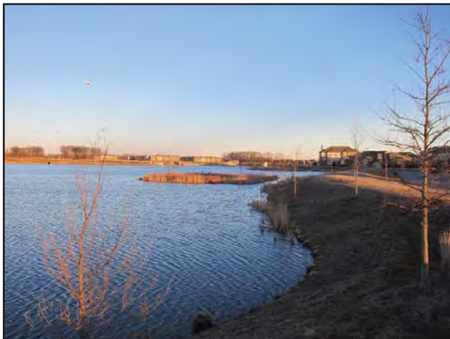
Detention facility at Saxony corporate campus in Noblesville
