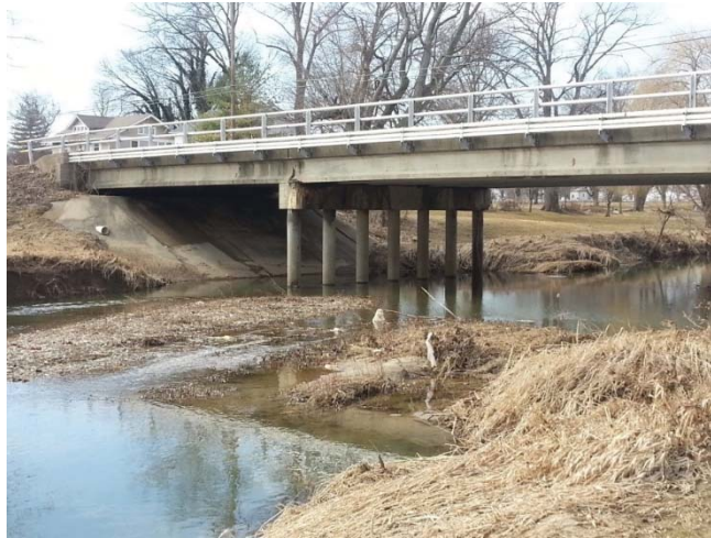
Photo 1: Sediment Accumulation Downstream of Main Street Bridge
