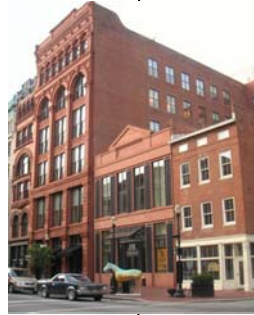
Historic windows have been repaired. New windows on infill structure harmonize with old.
