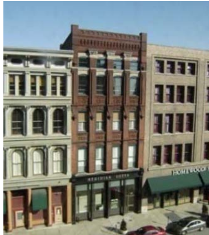
Contrast of missing and preserved cornice elements
