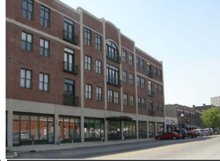
New building blends with four story buildings at other end of block in scale and with one story neighbor at street level by harmonizing window design and building materials.
