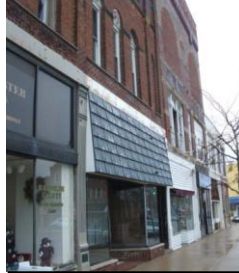
Inappropriate materials and use of Mansard roofing.
