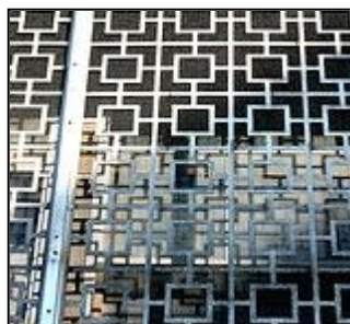
An example of inappropriate grillwork.
