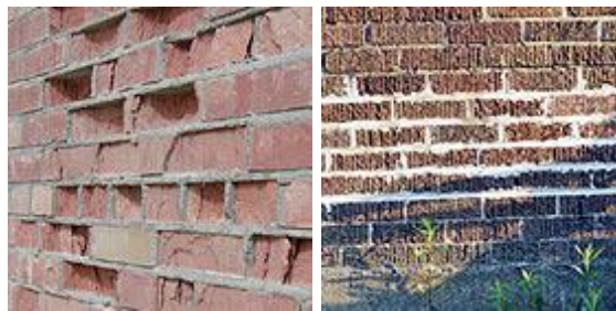
Excessively deteriorated brick
