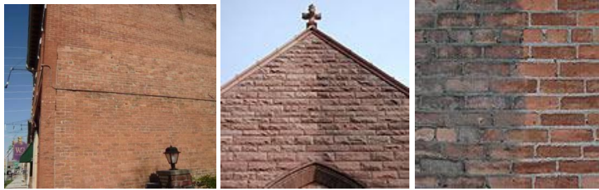
Examples of careful and appropriate cleaning
