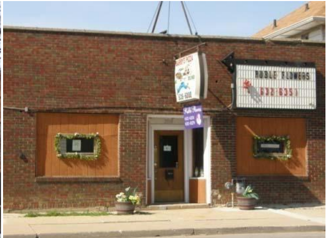
Filling in windows detracts from the architectural integrity of the building.
