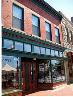
Transoms have been maintained with appropriate clear glass.
