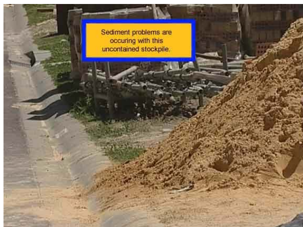
Sediment is the number one contributing pollutant from construction sites.
